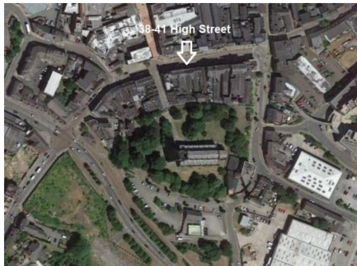
Figure 3.2 Frontage of 38-41 High Street
