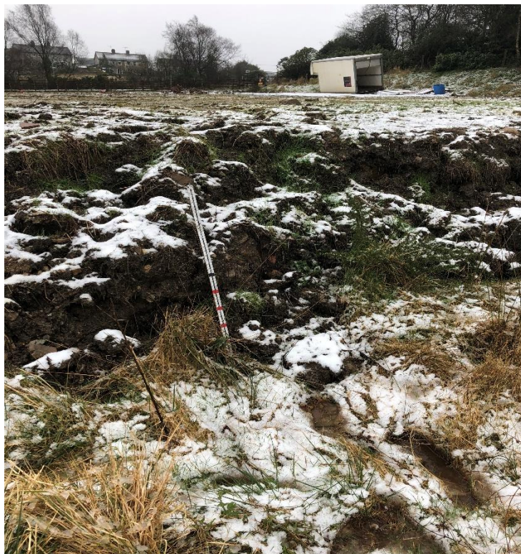
Photo 4 Infill thickness at Northern boundary
