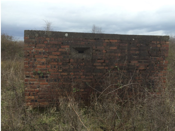
25- Typical pill box at site (B7)
