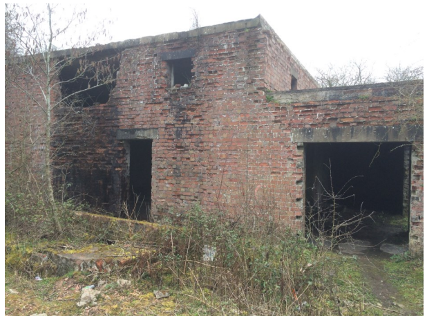
24- Exterior of Building 8
