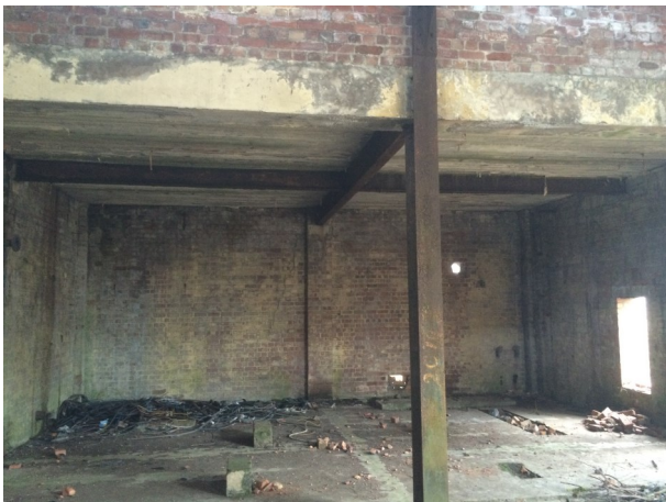
29- Interior of Building 3
