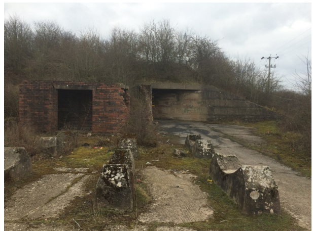
30- Exterior of Building 5 showing tunnel
