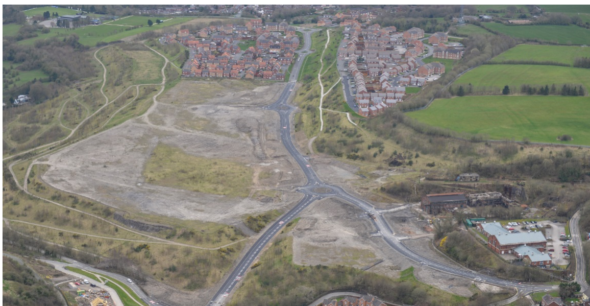
Figure 1: Image of the existing site – looking south
