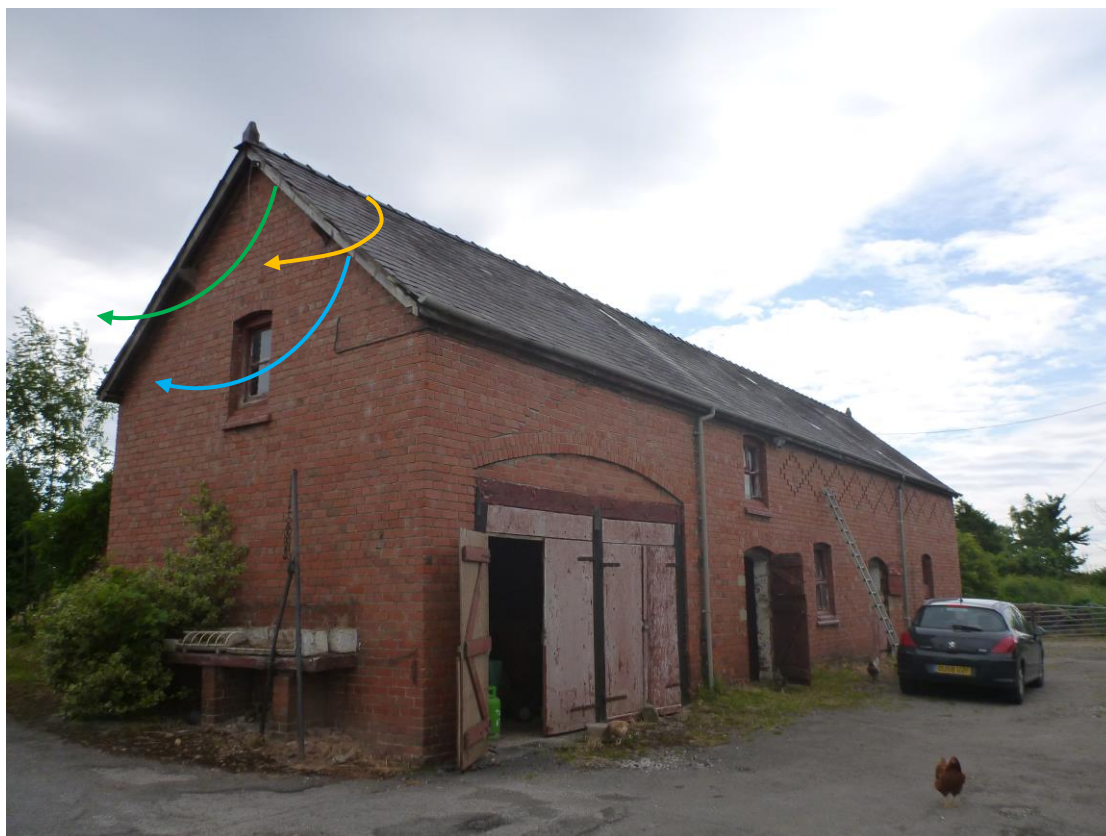
Figure 9. View from VP1 showing roost access points (one soprano pipistrelle, one indeterminate pipistrelle, and one whiskered bat).
