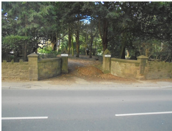
Existing Main Access
