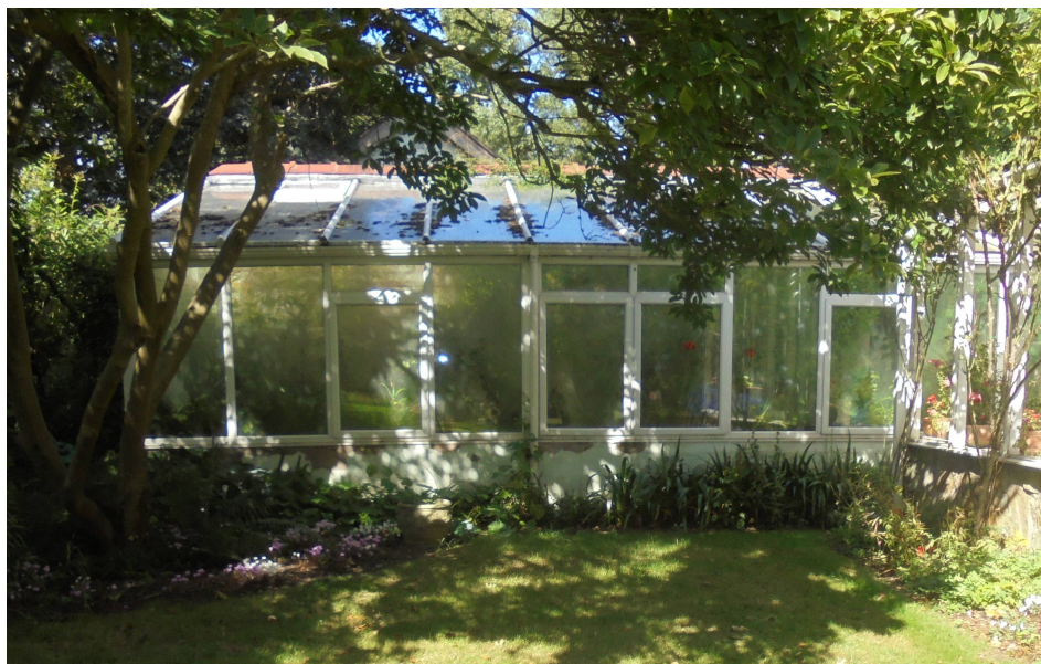
Existing Conservatory which is to be demolished
