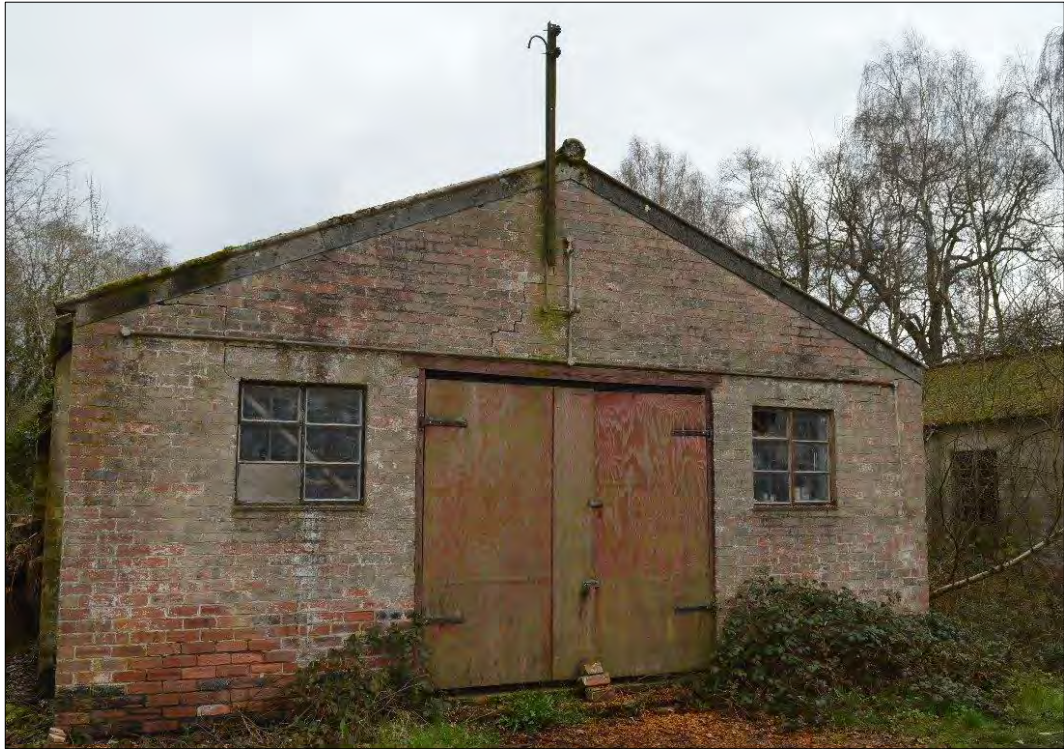
Fig. 7 West elevation of Building 1. Photo CPAT 4486-0085
