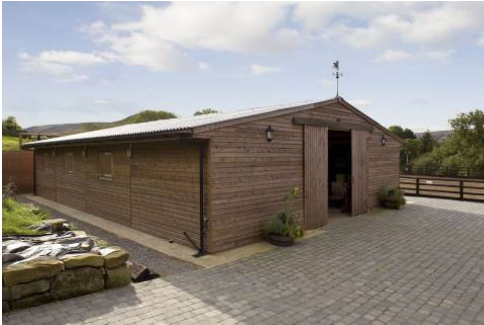
American barn with horizontal weatherboarding to the external face
