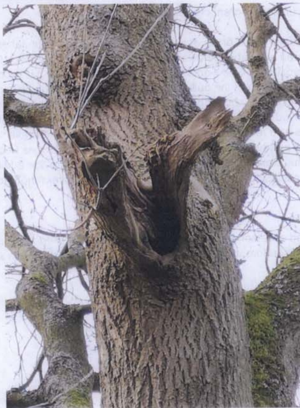
Figure 3: A photograph of the tear out within the large ash tree that sits just beyond the northern site boundary.
