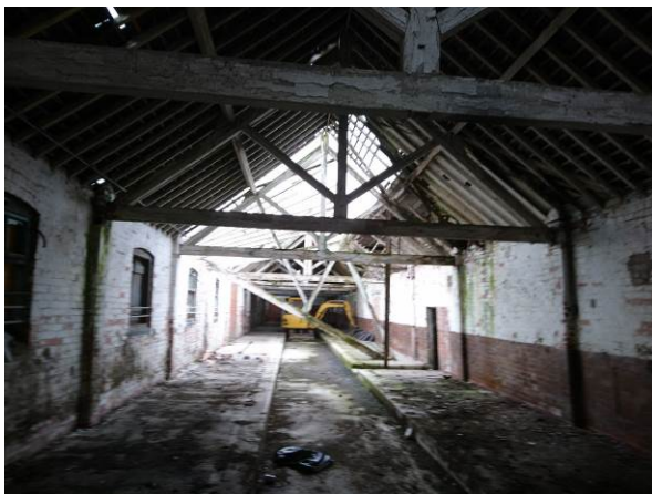
General view of roof over main part of building.
