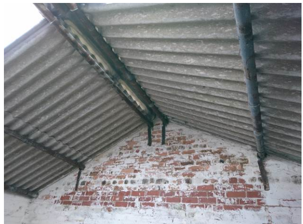
Typical construction of store roof.
