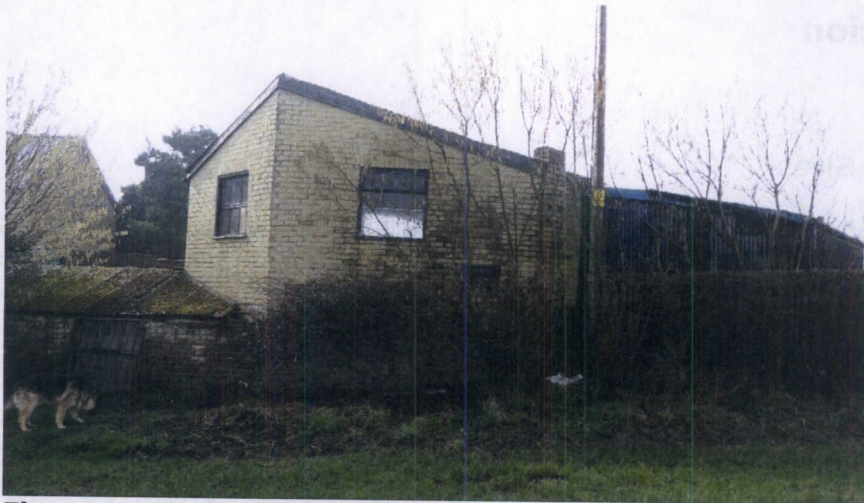
Figure 4.2 External view from north
