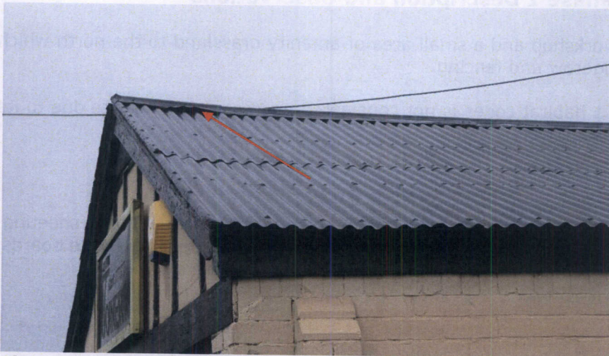
Figure 4.3 Potential access under roof ridge
