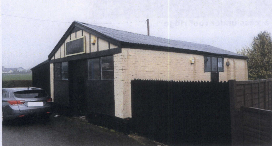
Figure 4.1 External view from south
