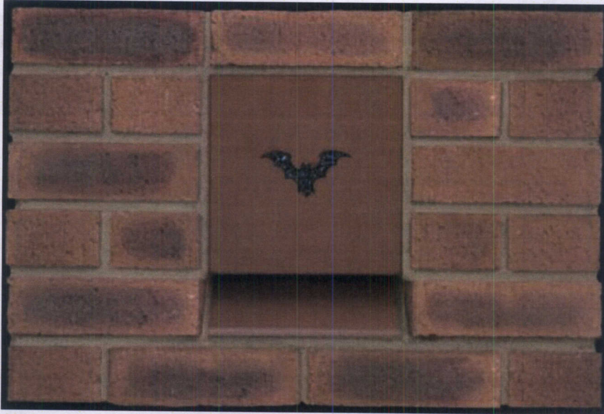
Figure 6.1. Integral bat box
