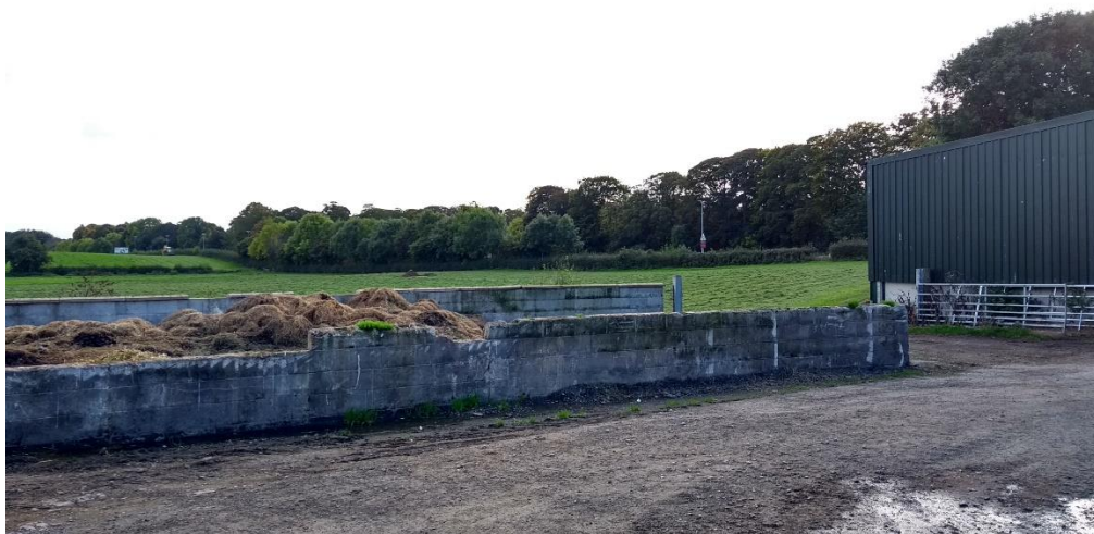
PLATE 2 – VIEW FACING NORTH TOWRDS STANSTY LODGE LANE
