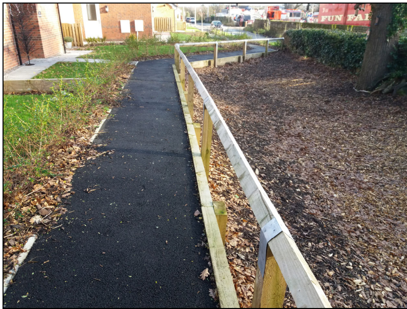
P1 & P2 – Example of completed no-dig footpath to be laid
