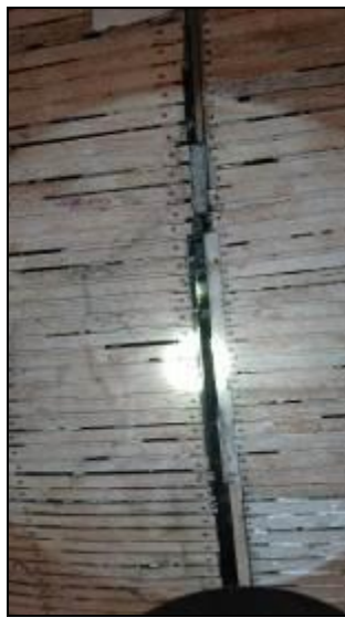
Plates 6-7 - The building interior upper floor (top) and gap in roof void visible (bottom)
