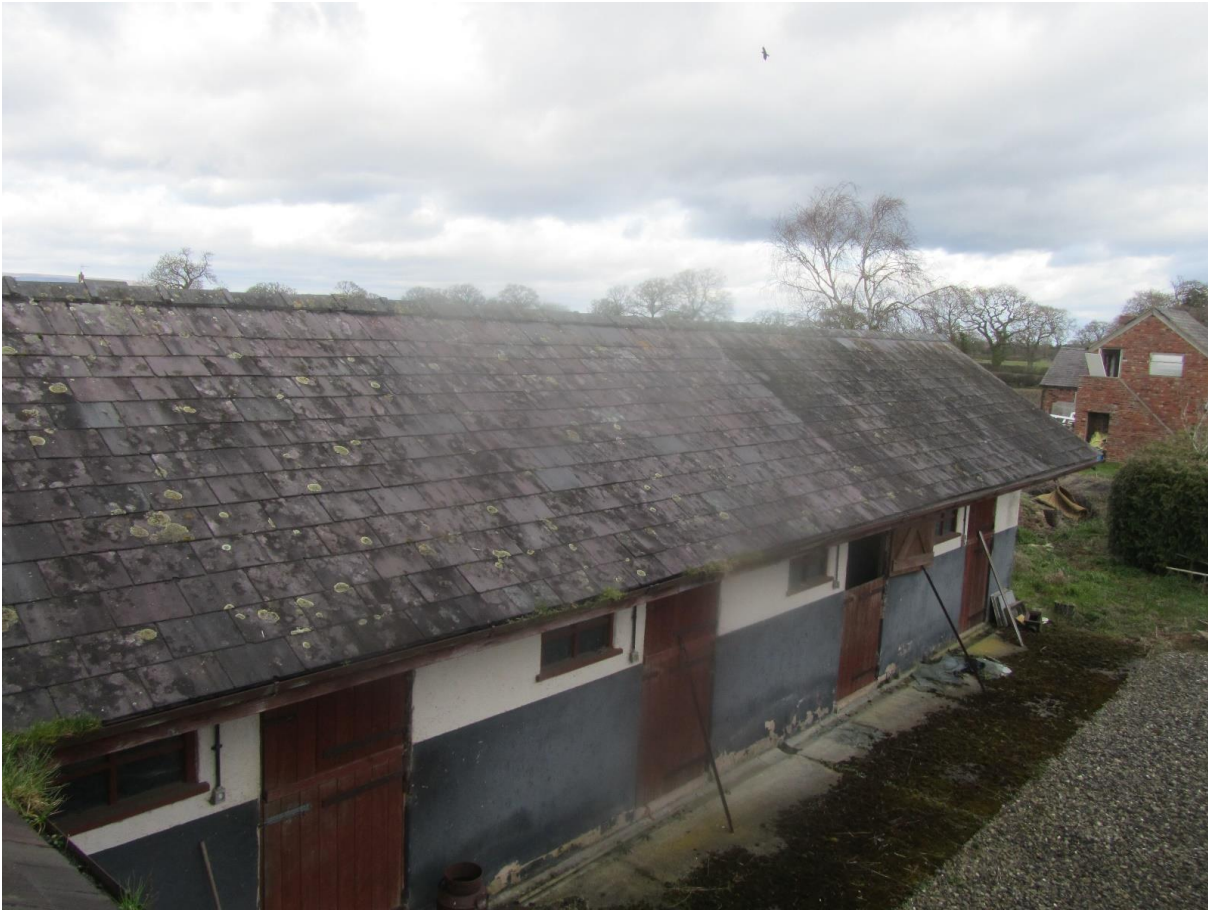
Image 21 A typical view of the roof of B3 (western-most stable block section)
