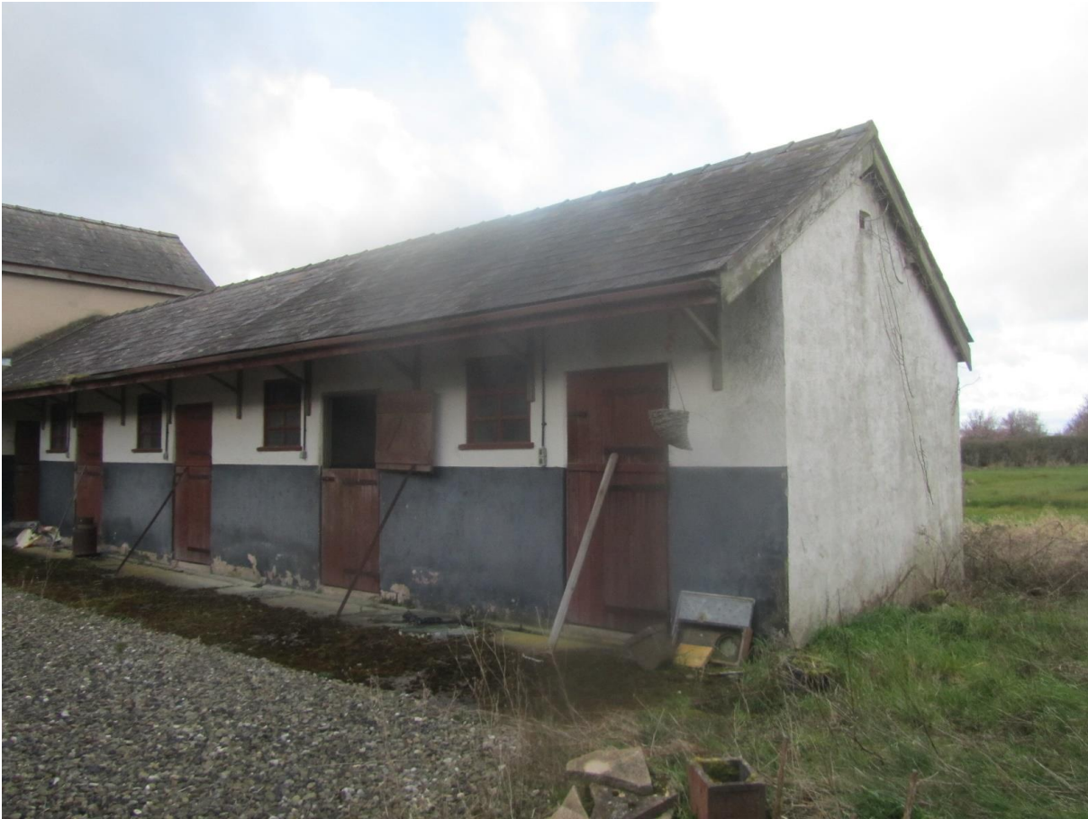
Image 15 Western-most stable block section of B3
