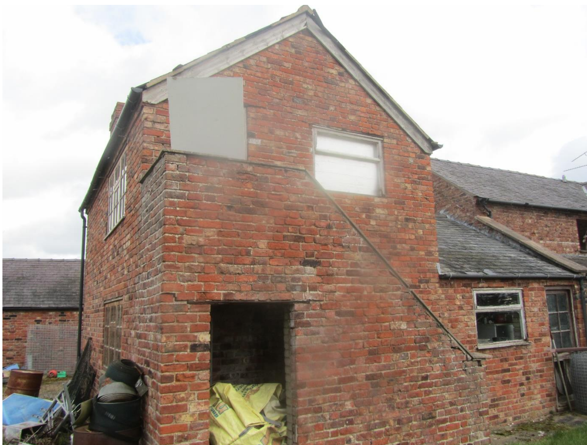
Image 10 southern and western elevations of B2
