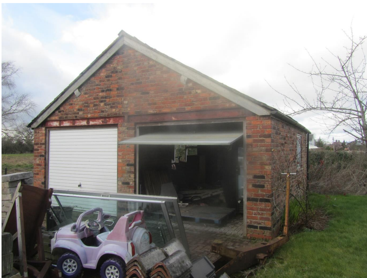
Image 2 Northern and eastern elevations of B1
