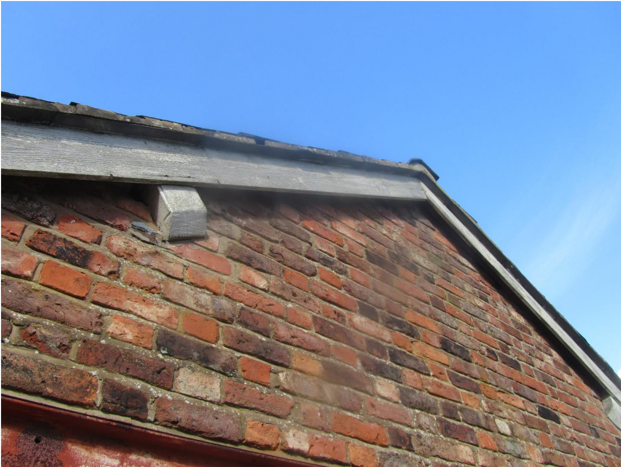
Image 3 Eastern gable end of B1
