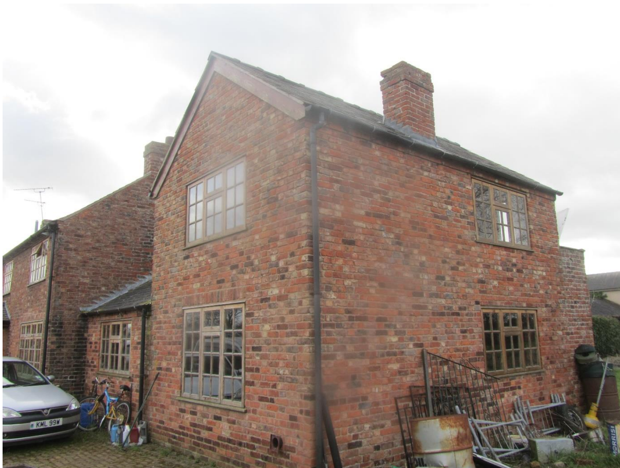
Image 9 Northern and western elevations of B2
