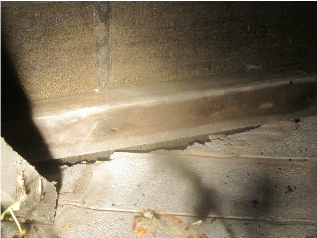
Image 22 Crevices between the timbers and internal eastern gable wall inside the barn section of B3
