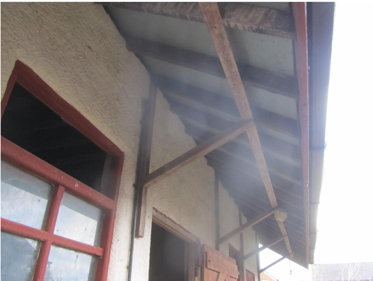
Image 18 Open eaves in the stable block sections of B3
