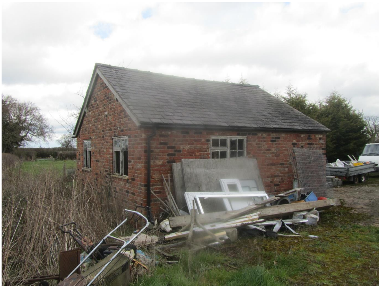
Image 1 Southern and western elevations of B1
