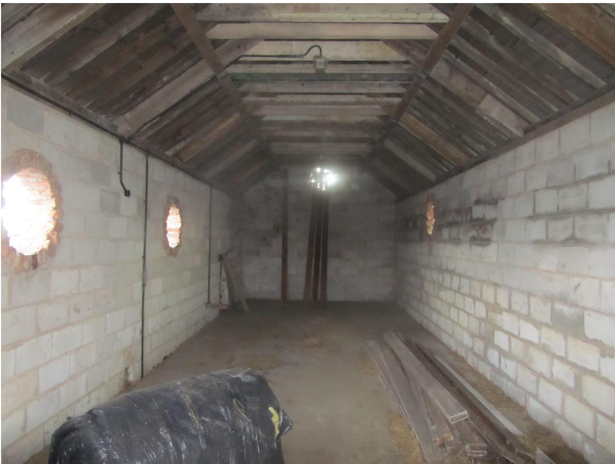
Image 20 A typical view within the barn section of B3 (first-floor)
