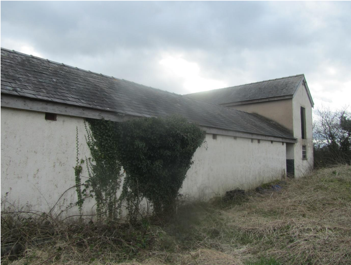
Image 17 Western elevation of B3, showing barn and stable block
