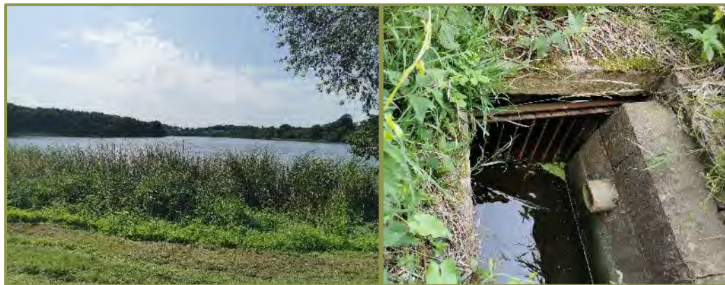
Left: Hanmer Mere Right: 1m x 1m Box Culvert to north of mere
