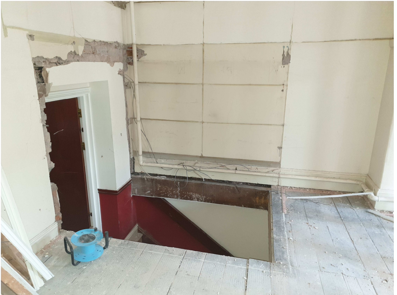
Photographs of Removal of Bulkhead to Ground Floor Staircase Proposed To Be Removed
