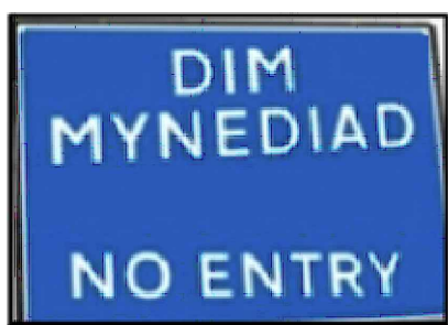
Signage fixed to the 2m High Steel Palisade Fence at the position of the removed entry/exit point
