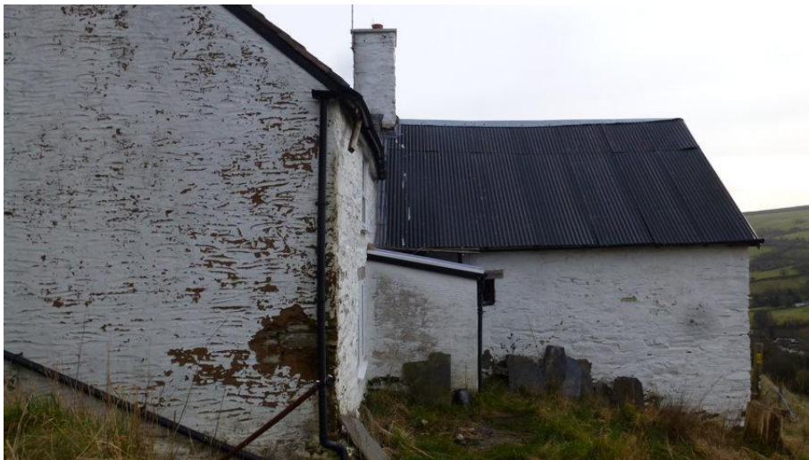
Photograph D: View of south facing frontage to building with corrugated metal roofing extension to rear.
