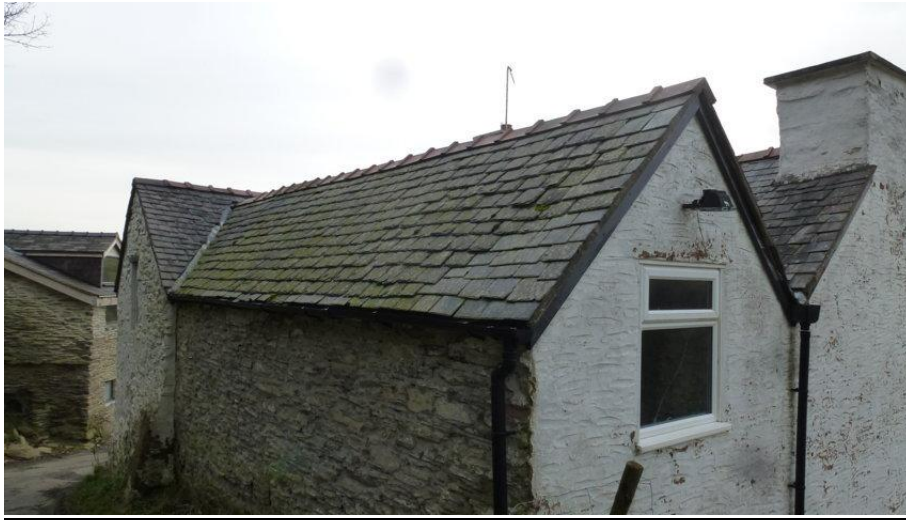
Photograph C: View of north facing frontage to target building.
