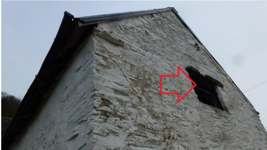
Photograph G: View of south facing gable end of barn structure with bat egress location via unglazed windows indicated.
