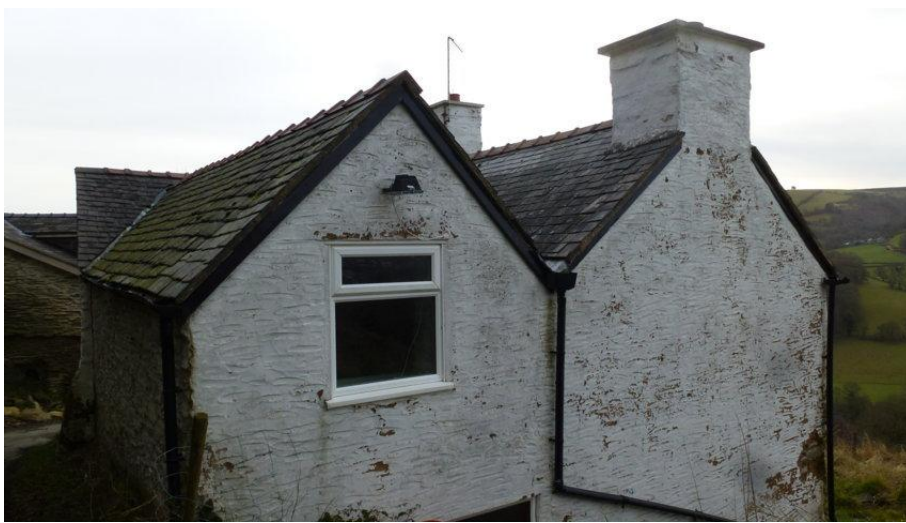
Photograph B: General view of rear (west facing) frontage to target building.
