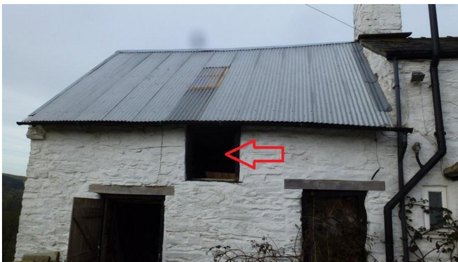
Photograph H: View of east facing frontage to barn structure with bat egress location via unglazed windows indicated.
