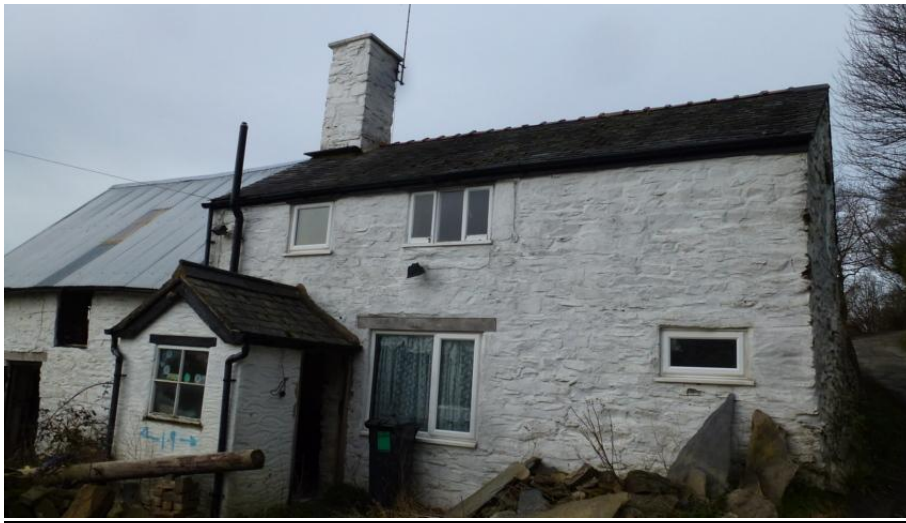
Photograph A: General view of front (east facing) frontage to target building.
