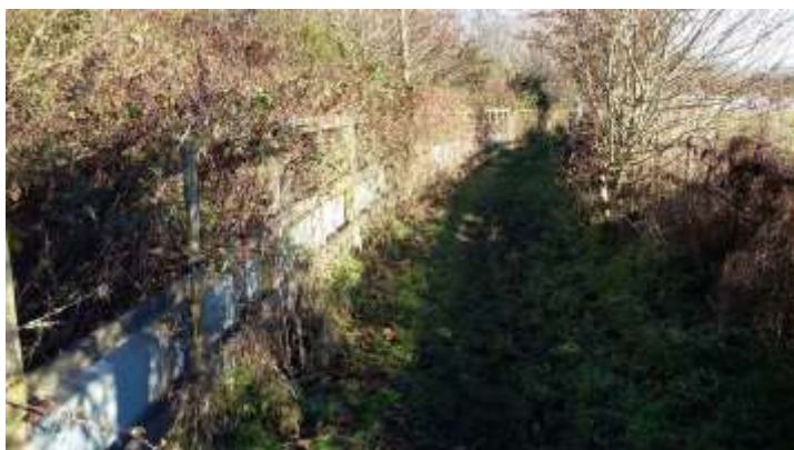
Plate 2. Showing intact exclusion fence but with unmanaged vegetation along northern boundary of Ty Cerrig
