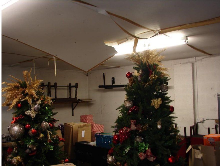
Internal view of garage (Target Note 4)
