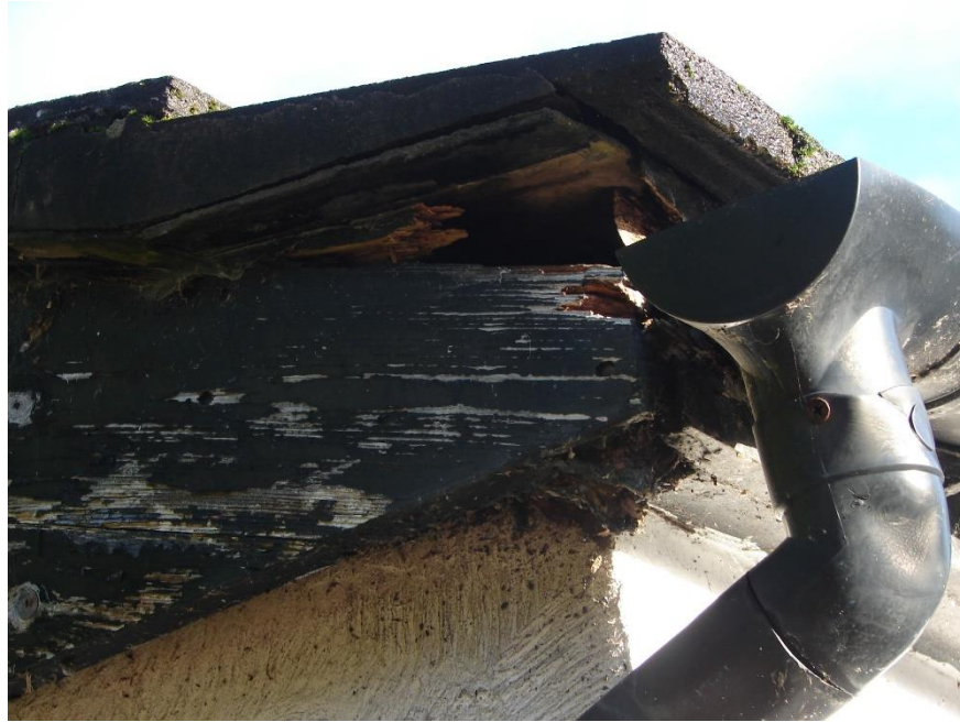
Hole in barge board, corner of Side C and Side D.
