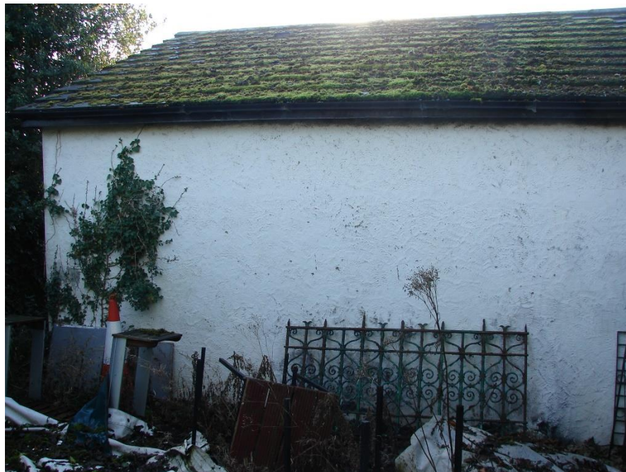
View of Side B. The roof tiles are in good condition.
