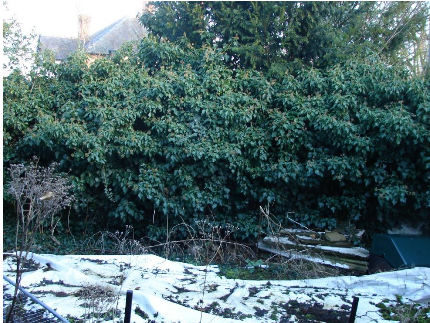
Part of the wall at Target Note 2 .
