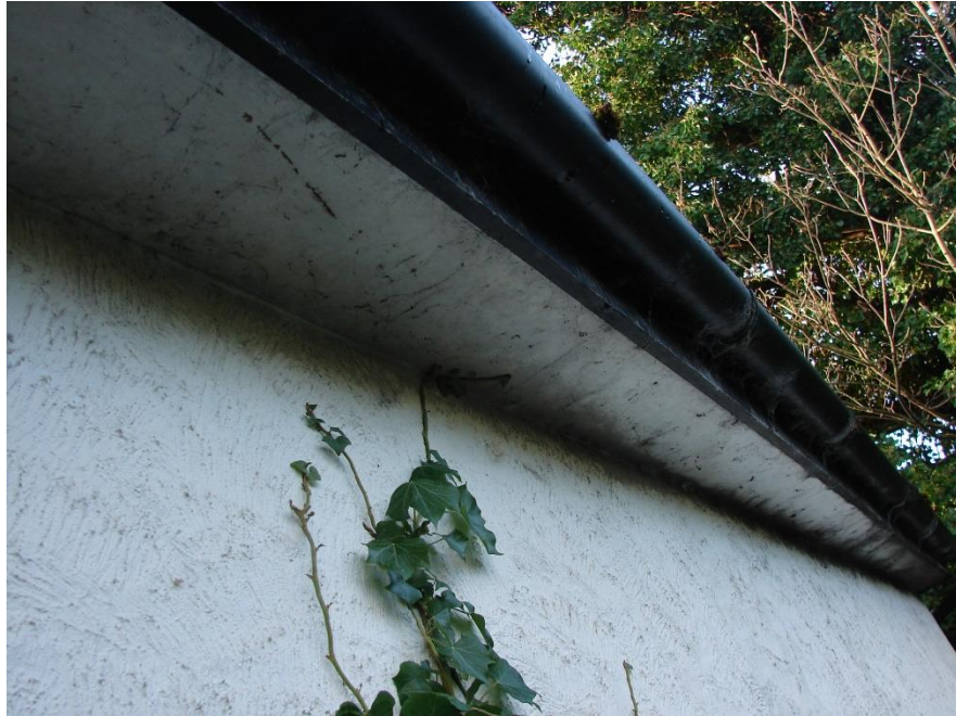
View of underside of soffit box on Side B. It is well sealed.
