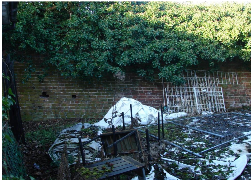
Part of the wall at Target Note 3 .
