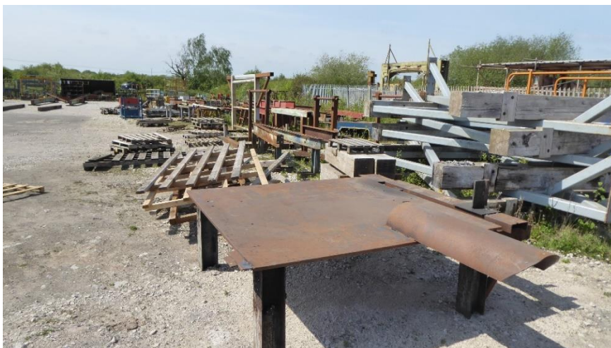
Figure 4.2 Stored materials along northwest
