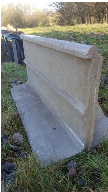
Figure 6.3. Example over-ground newt fencing section
