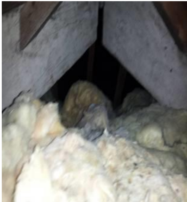
Interior of low level loft space over Mill cottage
