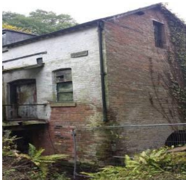
Adjoining mill and mill pit
