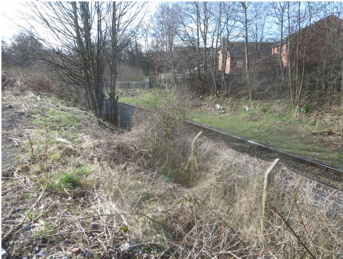
Image 3.4 A typical view of the western site margin and adjacent railway line, which will be retained and managed as the RCA (2018)
