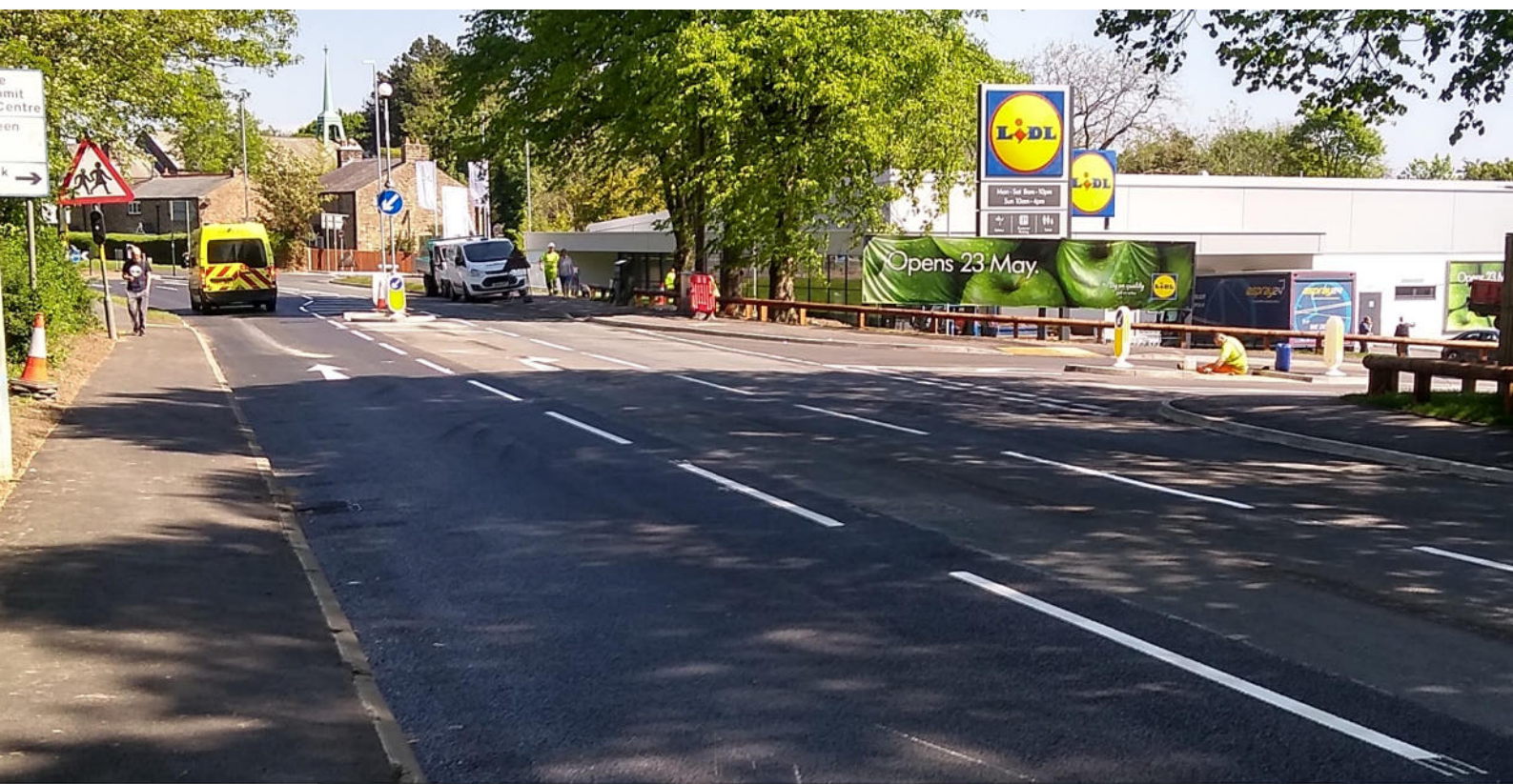
Above: Lidl at Clayton-le-Woods, Chorley, April 2019. Store and Section 278 works close to completion prior to opening
