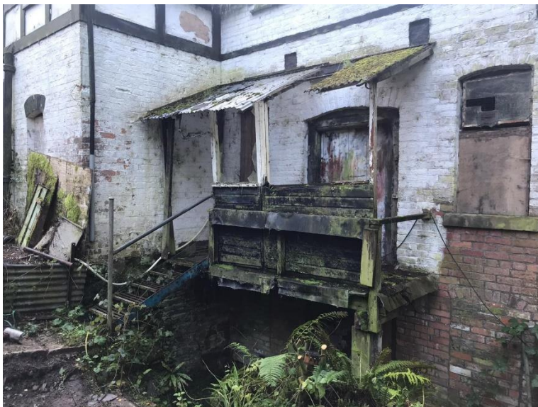
Existing porch, iron steps and balcony on north elevation
