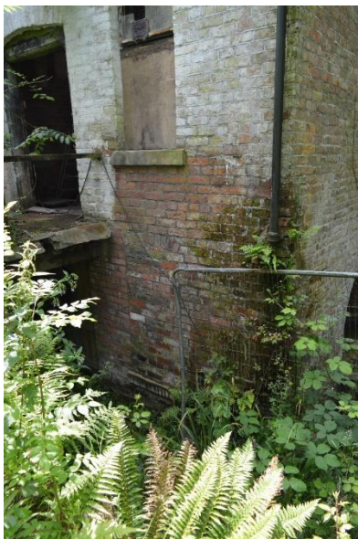
White paint weathered on brick
