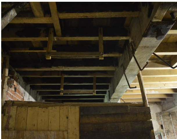
Cut/alterd joists in proposed kitchen area, showing portion of ceiling to be lowered
