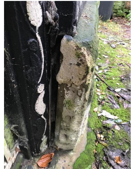
Stone plinth to be carefully removed where door is installed on south elevation and conditioned to stay on site
