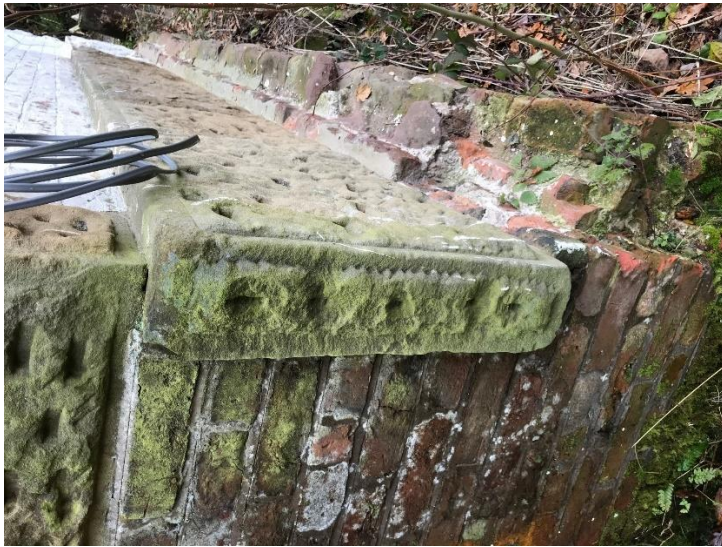
Stone plinth to be carefully removed where door is installed on south elevation and conditioned to stay on site
