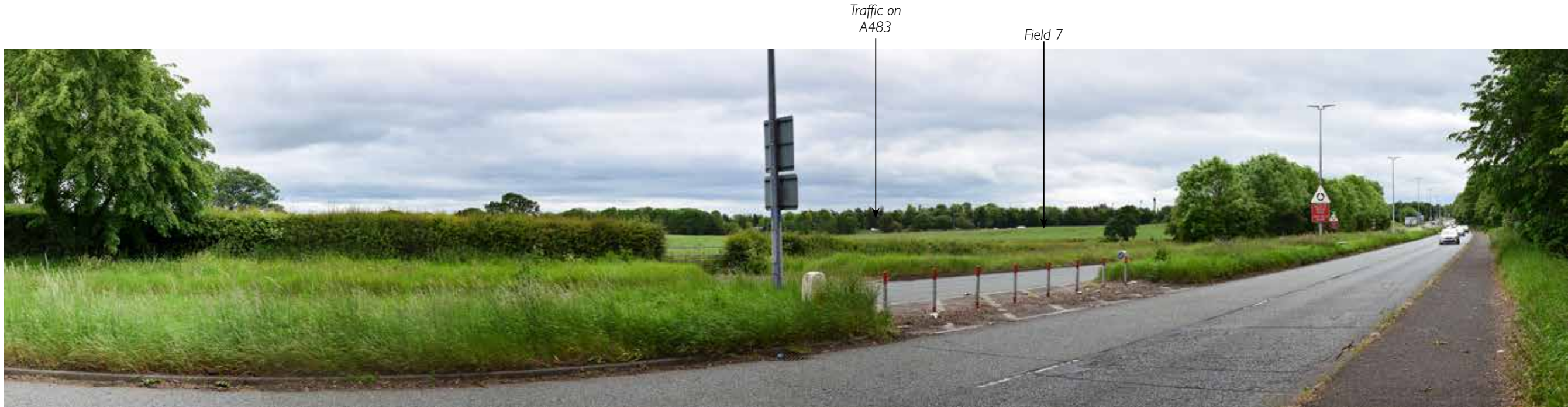
Photo 10.2 - View from A541 looking south east
