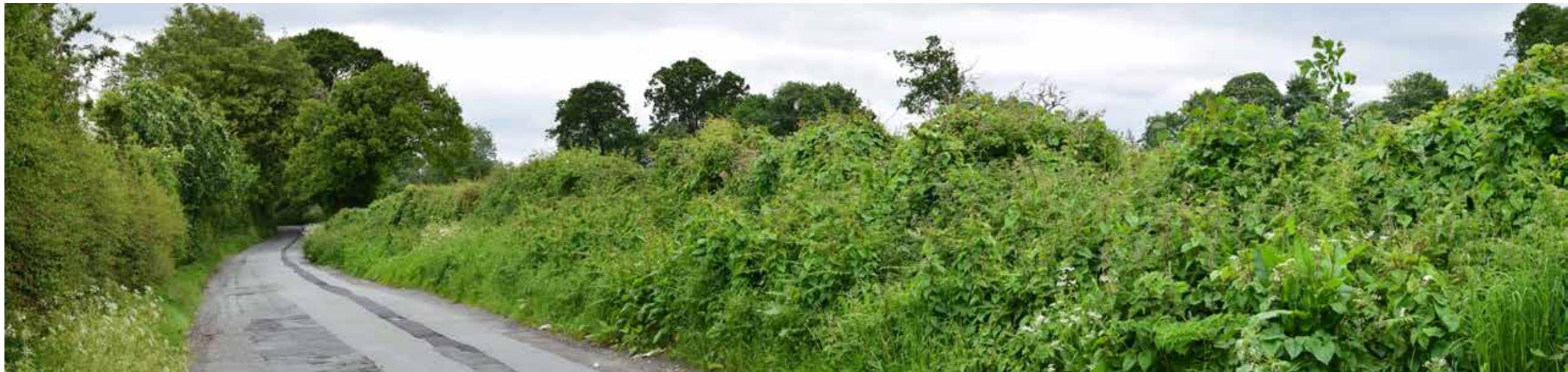
Photo 7.2 - View from Stansty Chain Road looking south east
