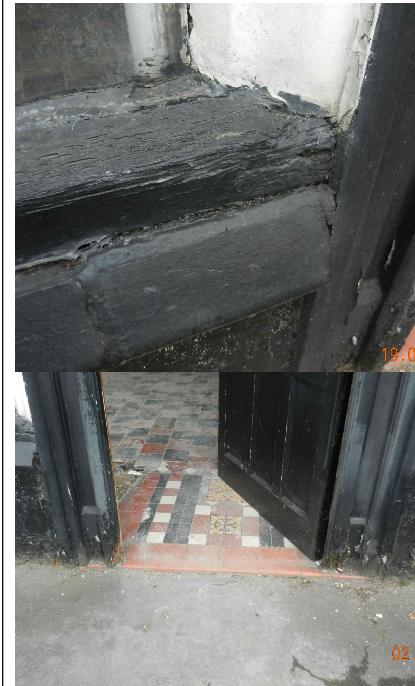
Images showing existing condition of shop front
