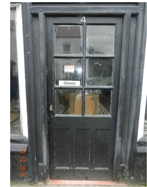
Image of existing main shop front door
