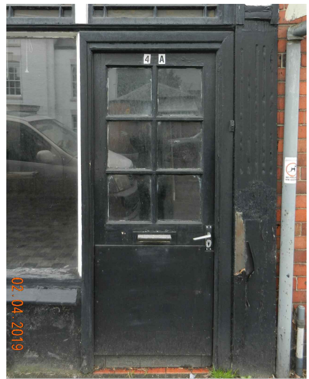
Image of existing right hand side shop door
