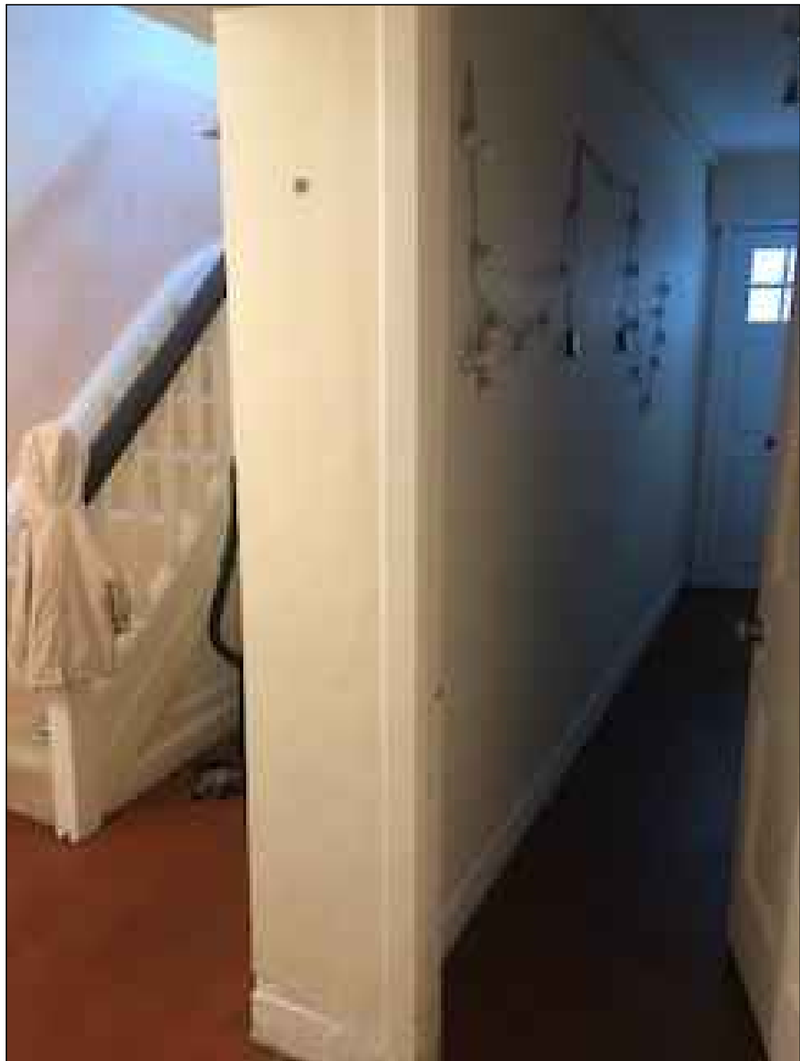
EXISTING VIEW ON OPENING 2.1 FROM HALL Scale 1:20
