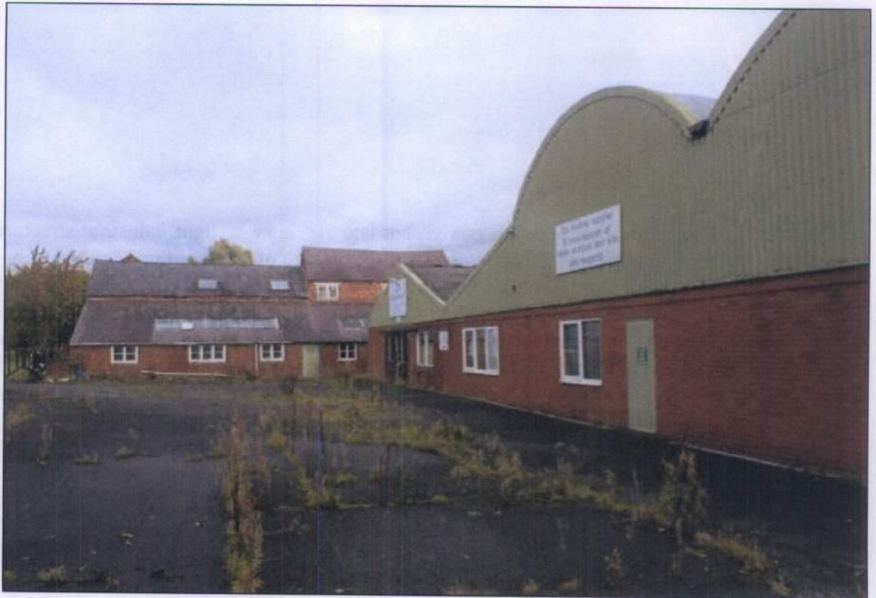
1. The application property, looking north towards the attached outbuilding of New Holt Lodge Farm
