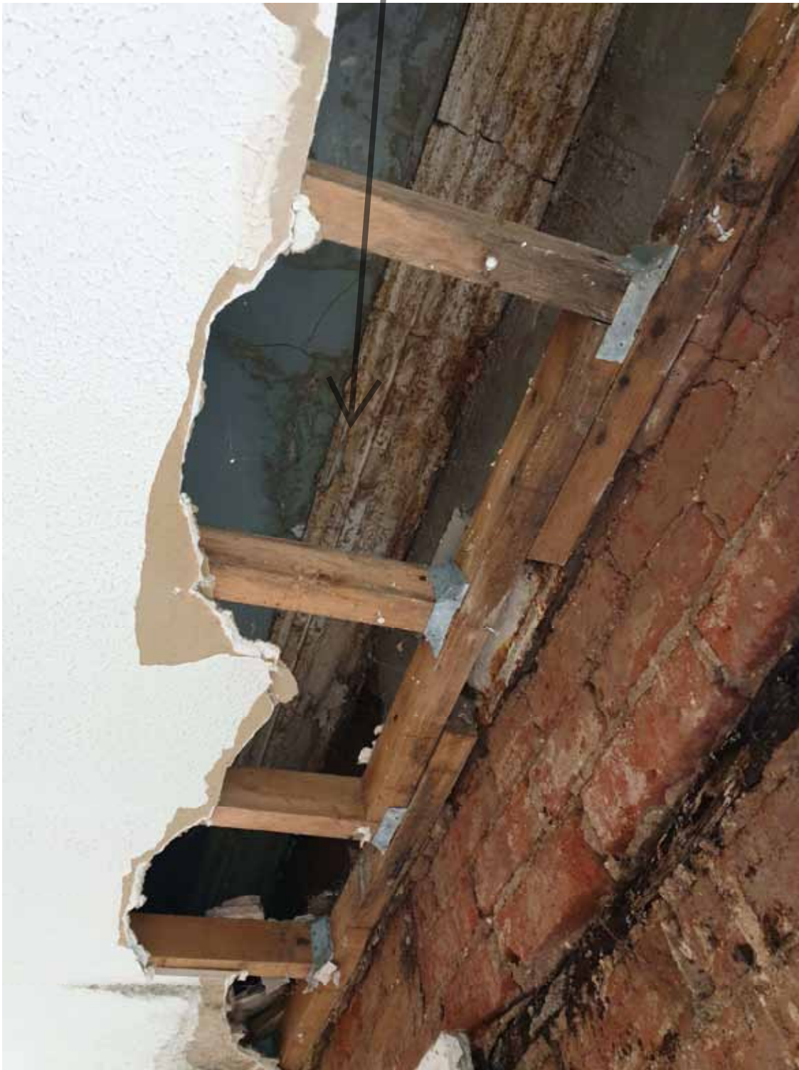
Photographs of Second Floor Suspended Ceiling & Roof Void To Frontage
