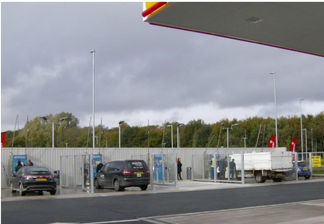
Jet wash bays Photo taken on handover day
