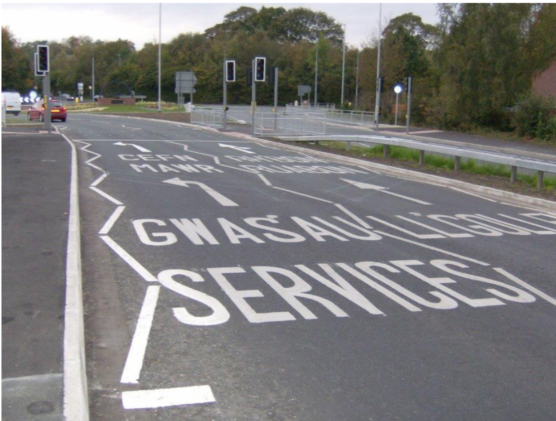
Road markings as part of s278 agreement
