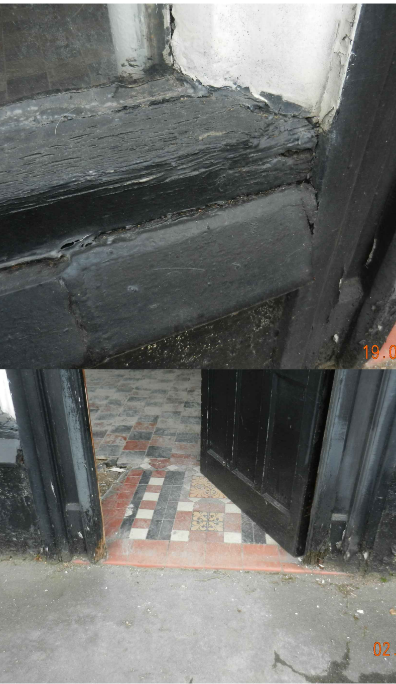
Images showing existing condition of shop front
