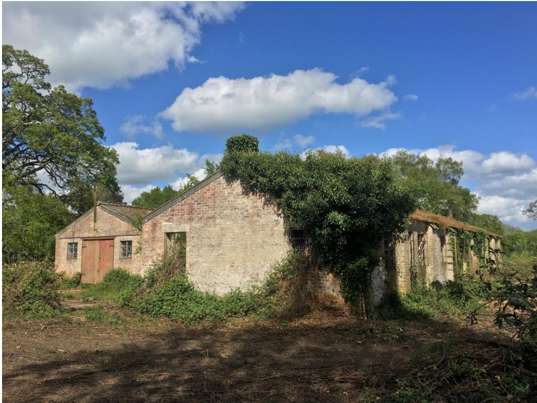
Fig. 1 Main brick building in south west corner of the Application Site
