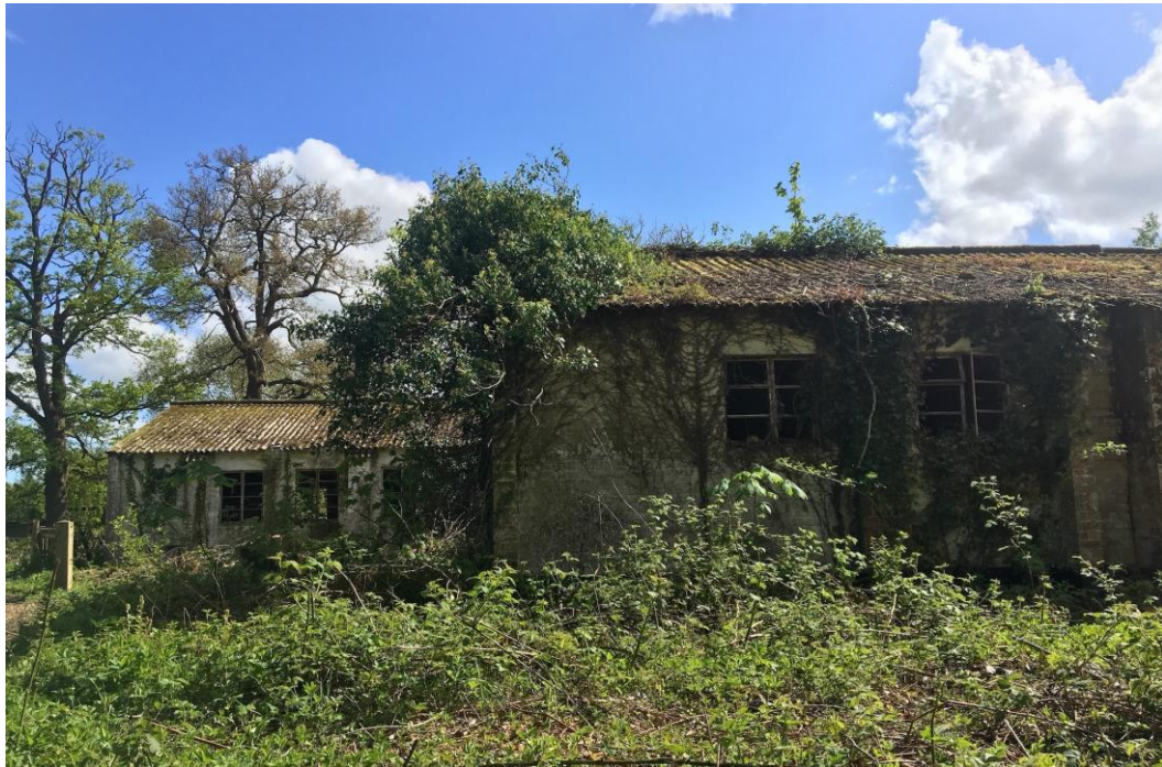
Fig. 5 South elevation of main brick building in south west corner of the Application Site
