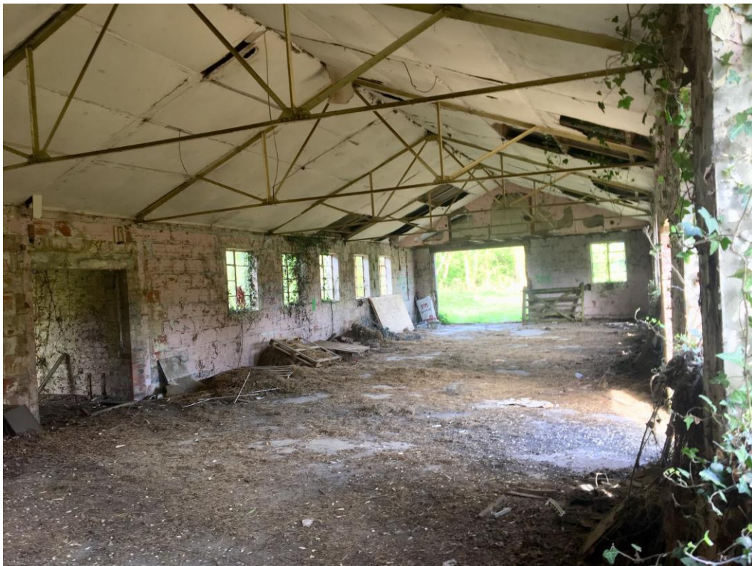
Fig. 6 Internal view facing East in main brick building
