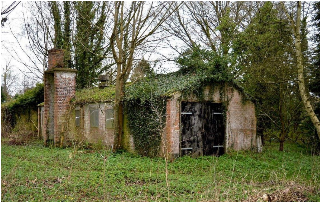
Fig. 7 Smaller brick building north east of the site, outside the Application area but within the Applicants ownership
