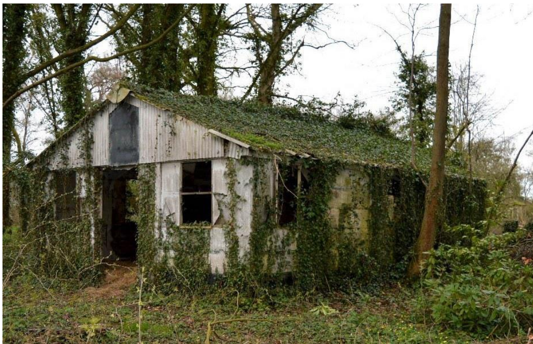
Fig. 8 Metal clad framed building in the eastern section of the Application Site
