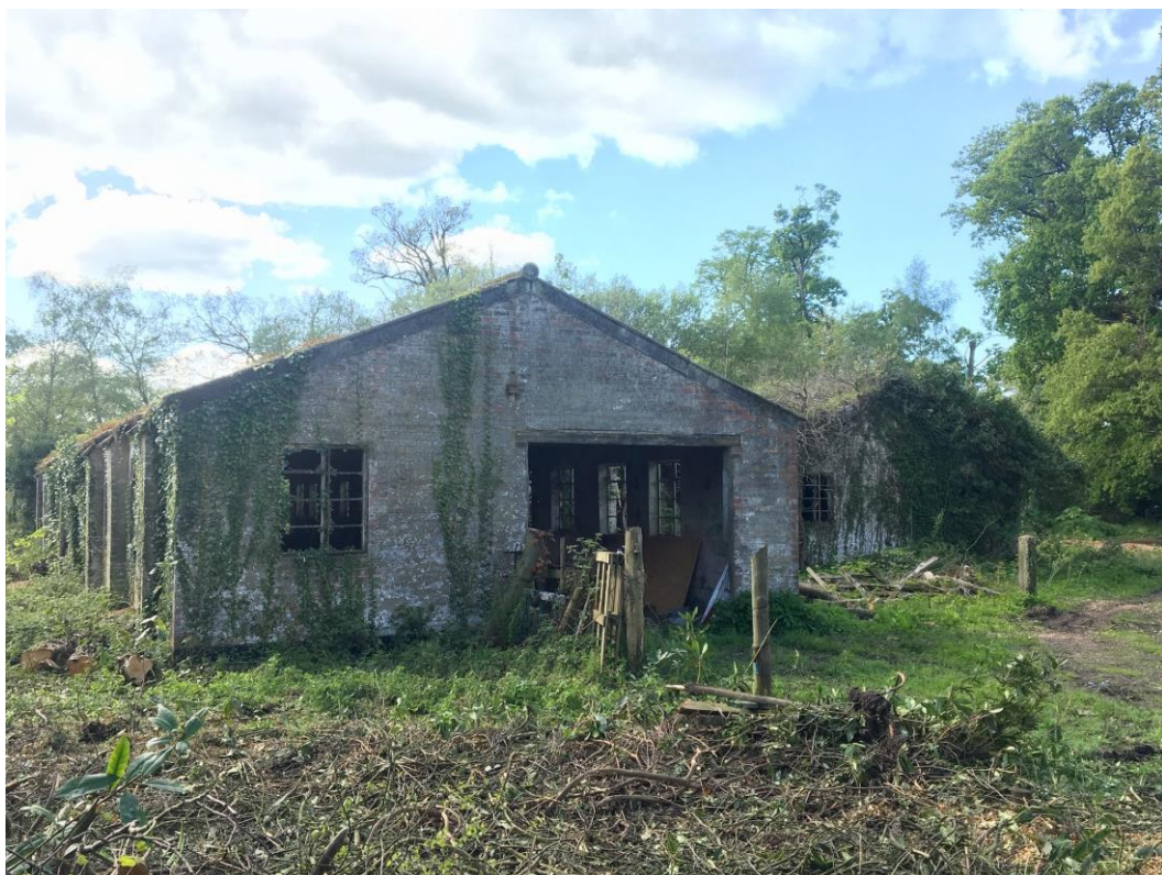
Fig. 4 East elevation of main brick building in south west corner of the Application Site
