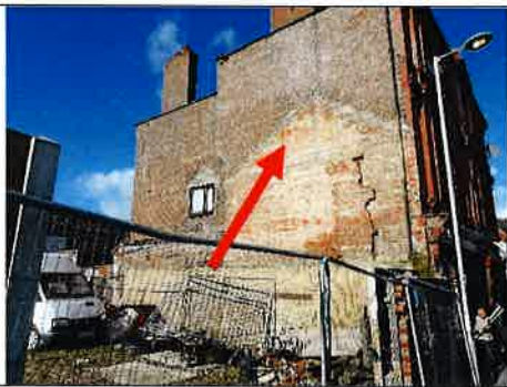
Fig 12- side denoting previous outline of building
