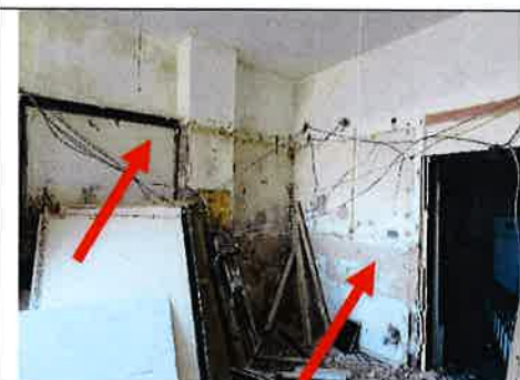
Fig 7- external and internal walls
