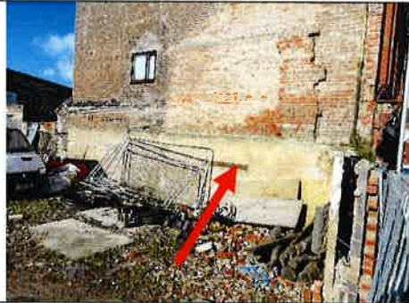
Fig 13- cement based render
