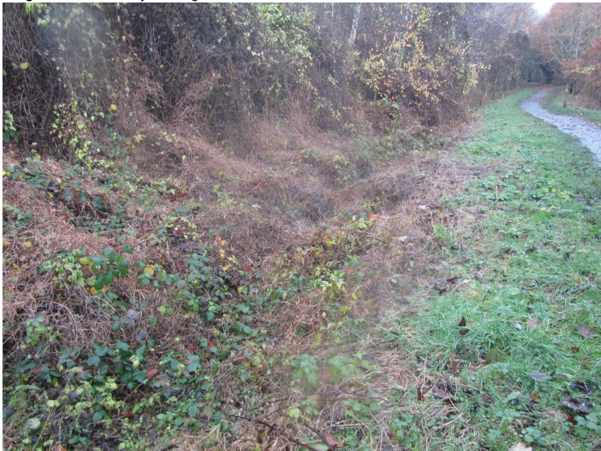
Image 3.16 WB2 – a dry and vegetated ditch
