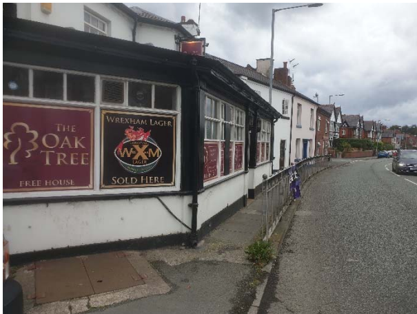
This photograph indicates the location of the existing barrel drop to be filled in and tarmacked over.
