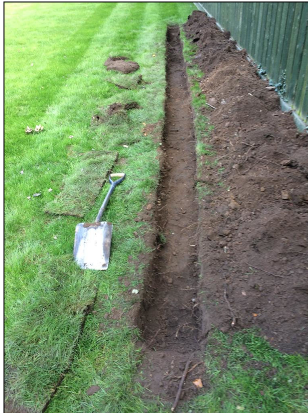
Photo 1 – Trench hand excavated to 300mm showing no significant roots
