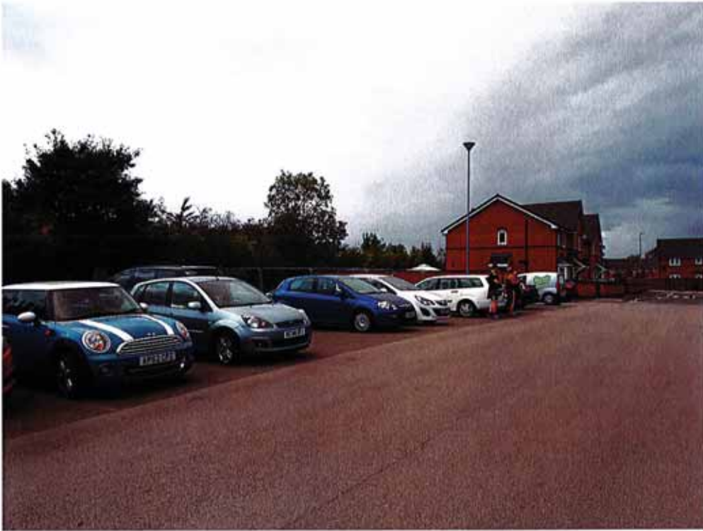
Photograph 3 Western section of the site from the south
