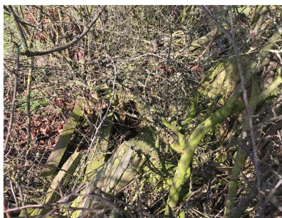
Photograph of T4 failure
