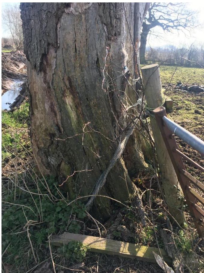
Photograph of T1 showing extensive decay
