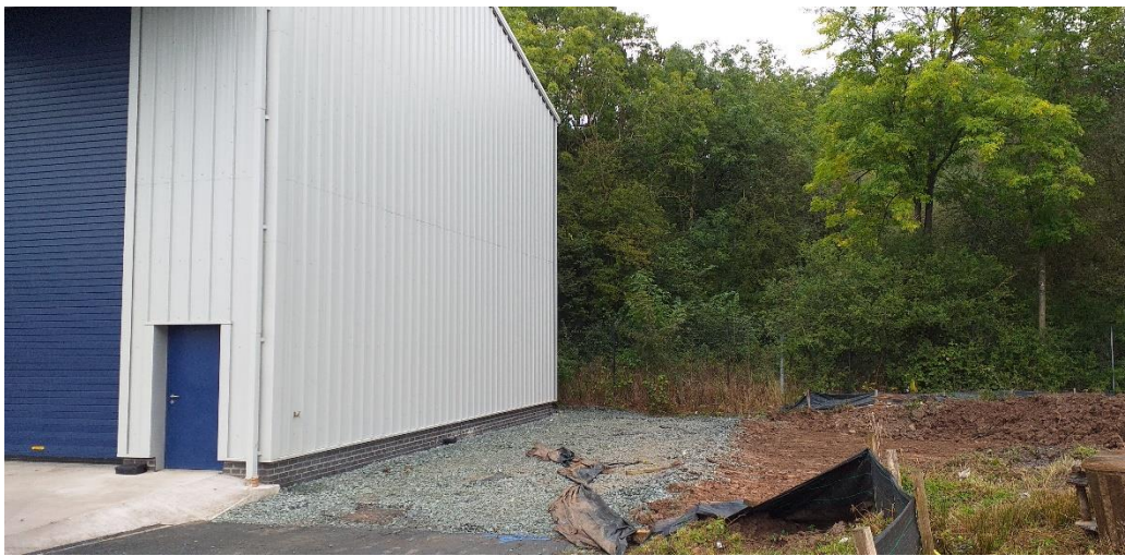
PHOTO 4.1 – LOCATION OF NEW PROPOSED EXTENSION TO THE EAST OF THE STORAGE SHED
