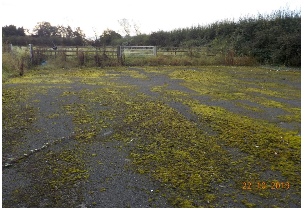
Plate 1: View looking at area hard standing at site entrance
