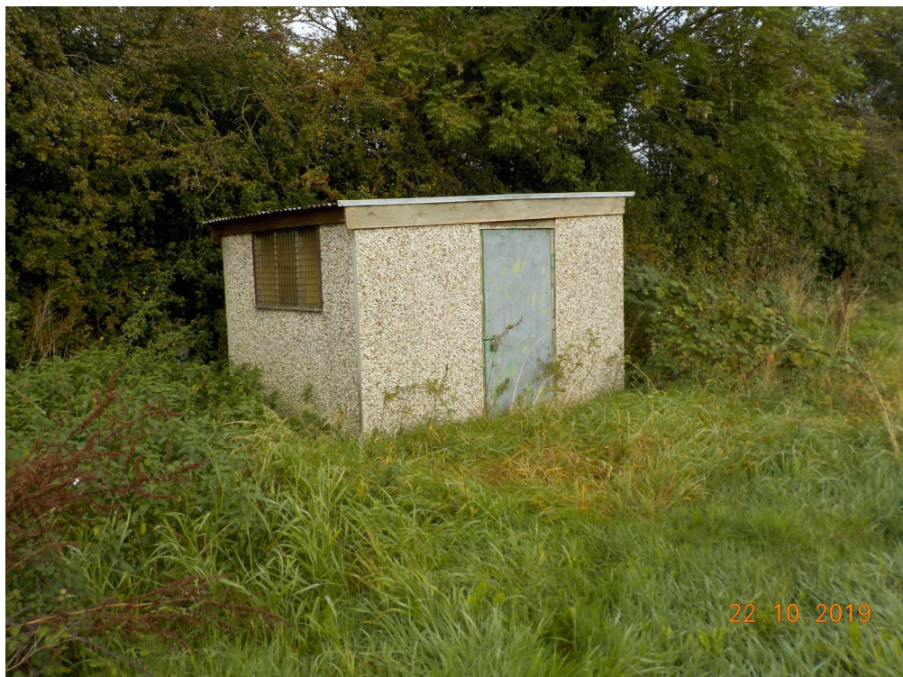
Plate 8: View of Building 1
