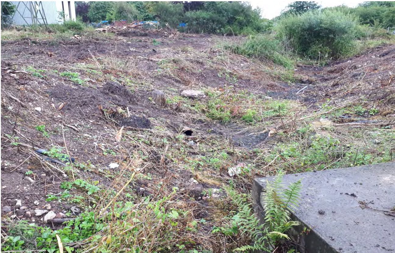
View East: Gully leading from concrete service cover. Drainage pipe exposed in northern gully face
