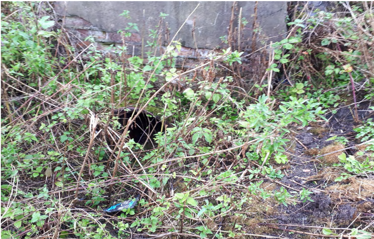
Drainage pipe in eastern face of concrete service cover
