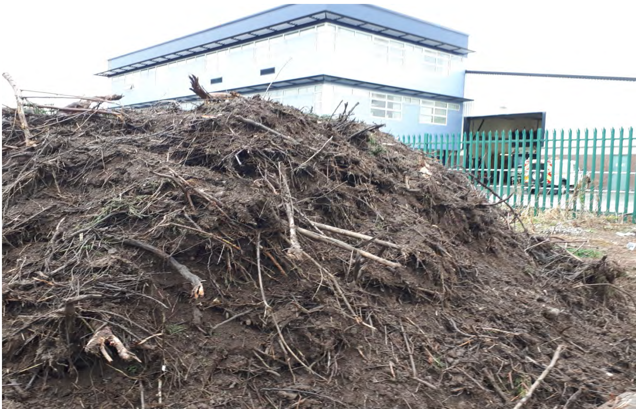
View North West of spoil heap created during site clearance
