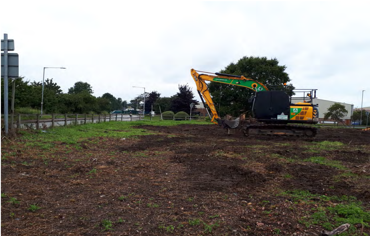
View West along southern site boundary
