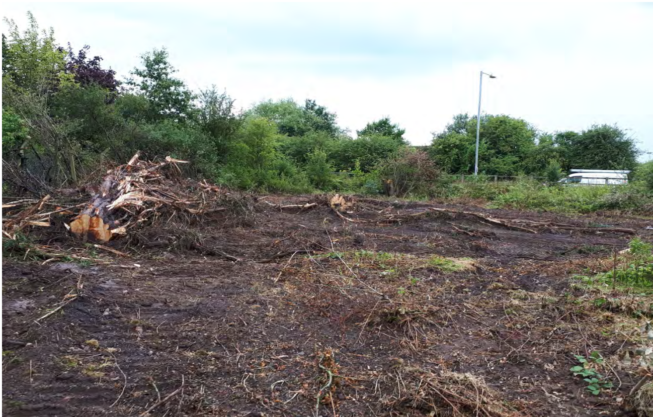
View South along eastern site boundary
