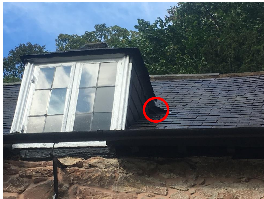
Plate 2: Roost 2, raised lead flashing retained
