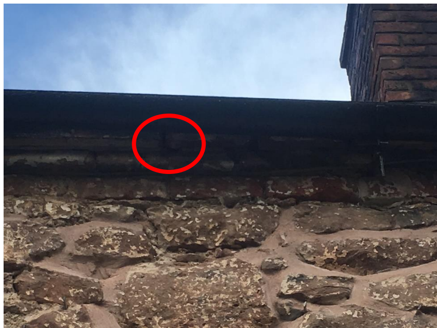
Plate 1: Roost 1 retained below guttering
