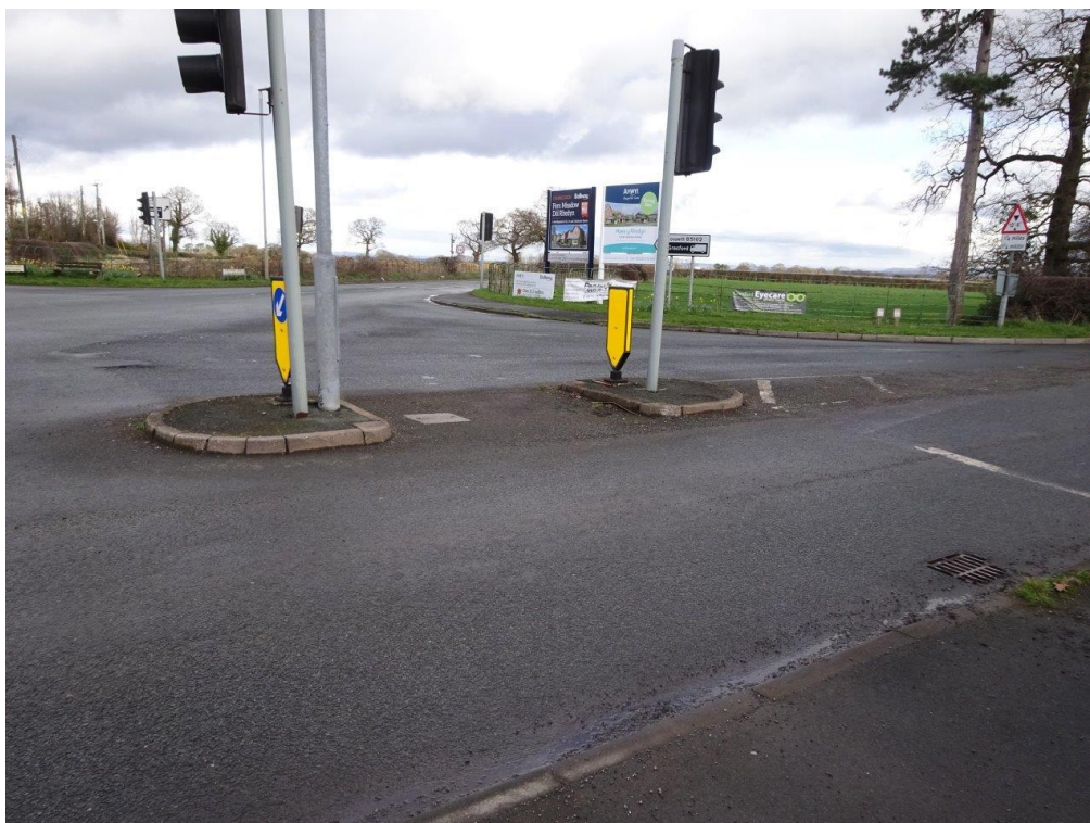
13.5 Crown Crossroads – Lack of pedestrian facilities
