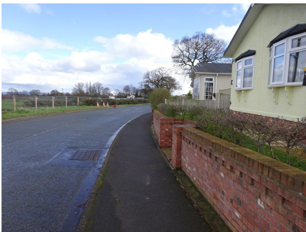
13.2 Gresford Road Puffin – Reduced visibility from southwestern footway
