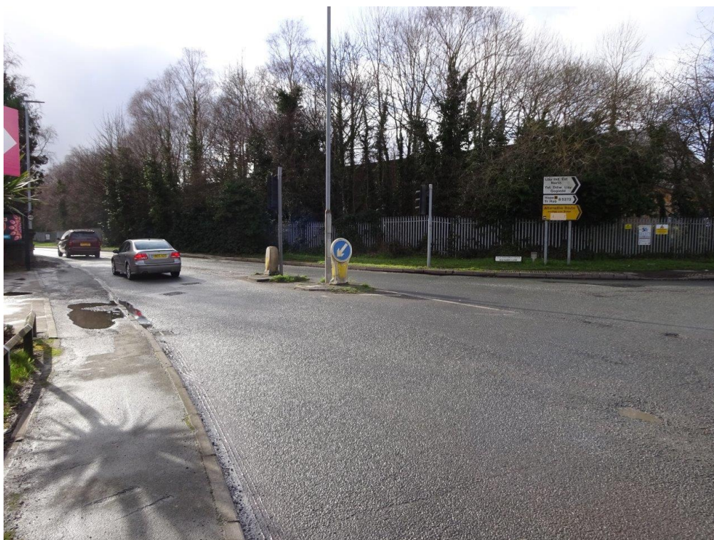
13.4 Crown Crossroads – Lack of pedestrian facilities
