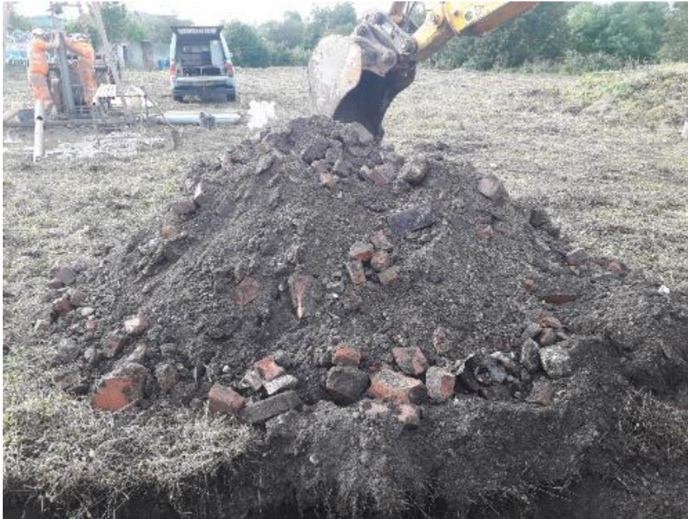
Plate 2: Trial Pit 1 – spoil
