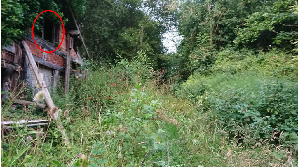
Figure 6: Emergence point of common pipistrelle and lesser horseshoe bat at the outbuilding to the north-east
