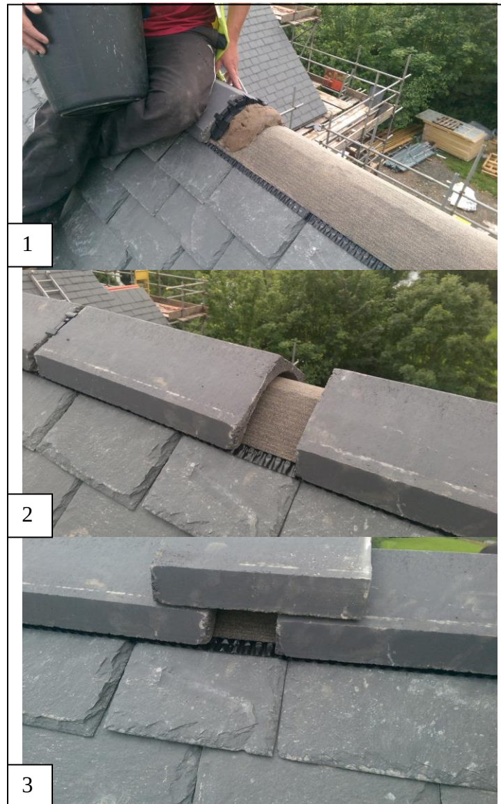
Figure 10: Indicative ridge tile access specification
