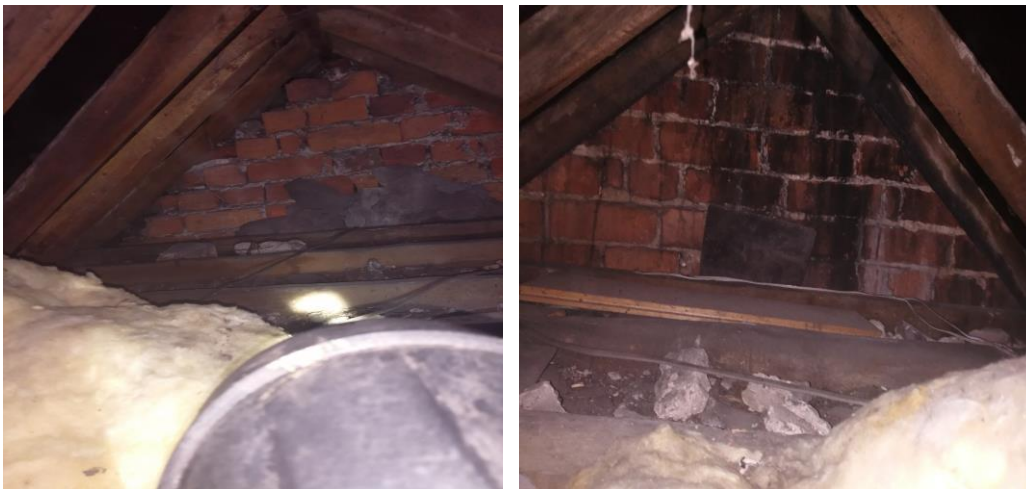
Plate 4: Accessible areas of loft space within Mill Cottage
