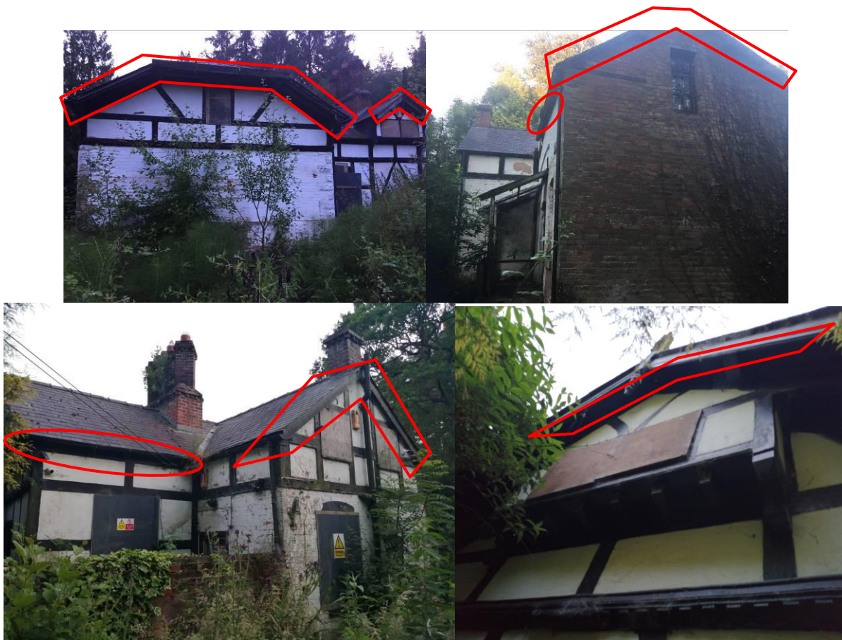
Figure 5: Emergence points at Mill Cottage indicative
