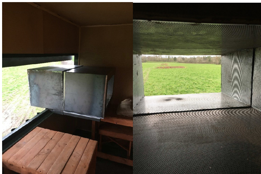
Figure 6.1: Images of Constructed Baffles (2 No. Boxes)
