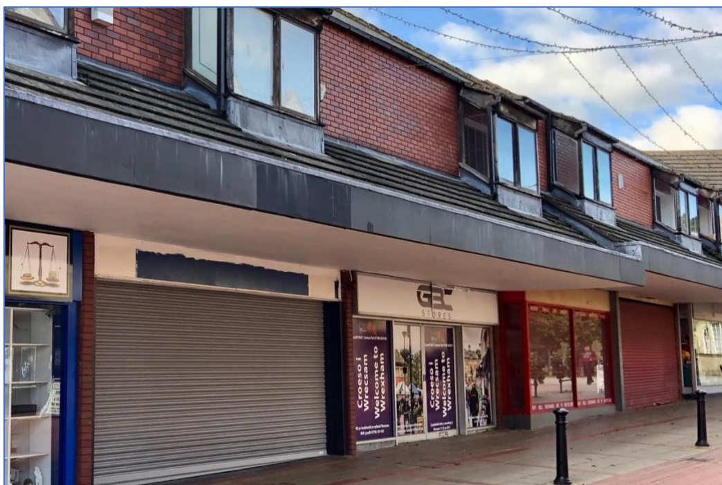
Photo 6 – Fronting Queen Street
