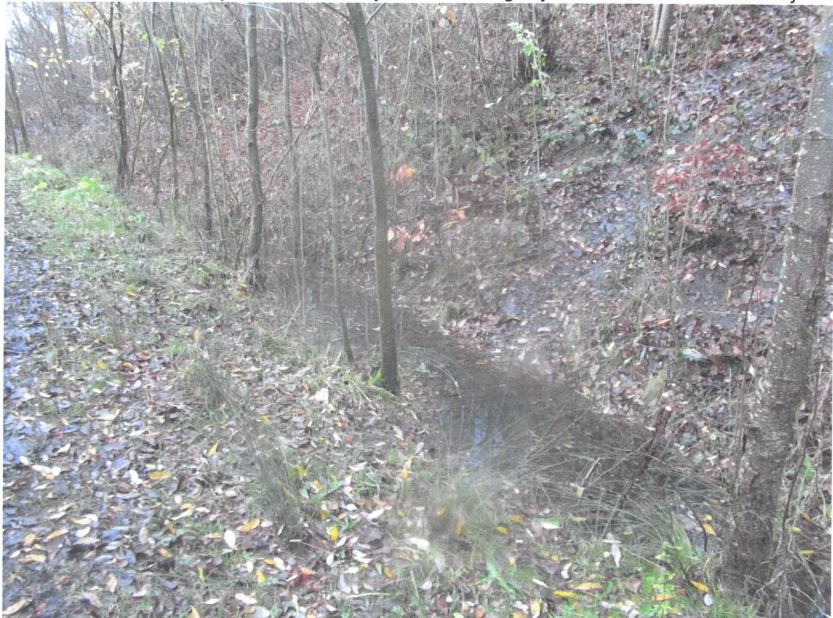
Image 3.21 WB7 – the only ditch/ drain surveyed to be holding any water at the time of the survey
